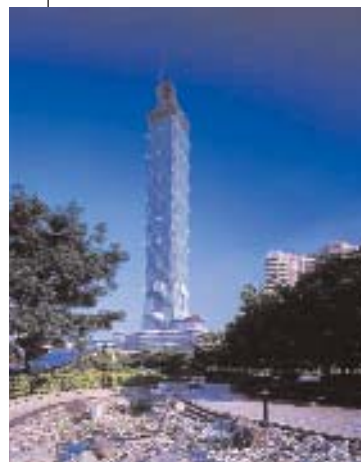
Facing and above: the Taipei finance tower is designed to resemble a growing bamboo shoot or an inverted pagoda. Inclining four degrees inwards, the structure increases in size as it gets higher.
